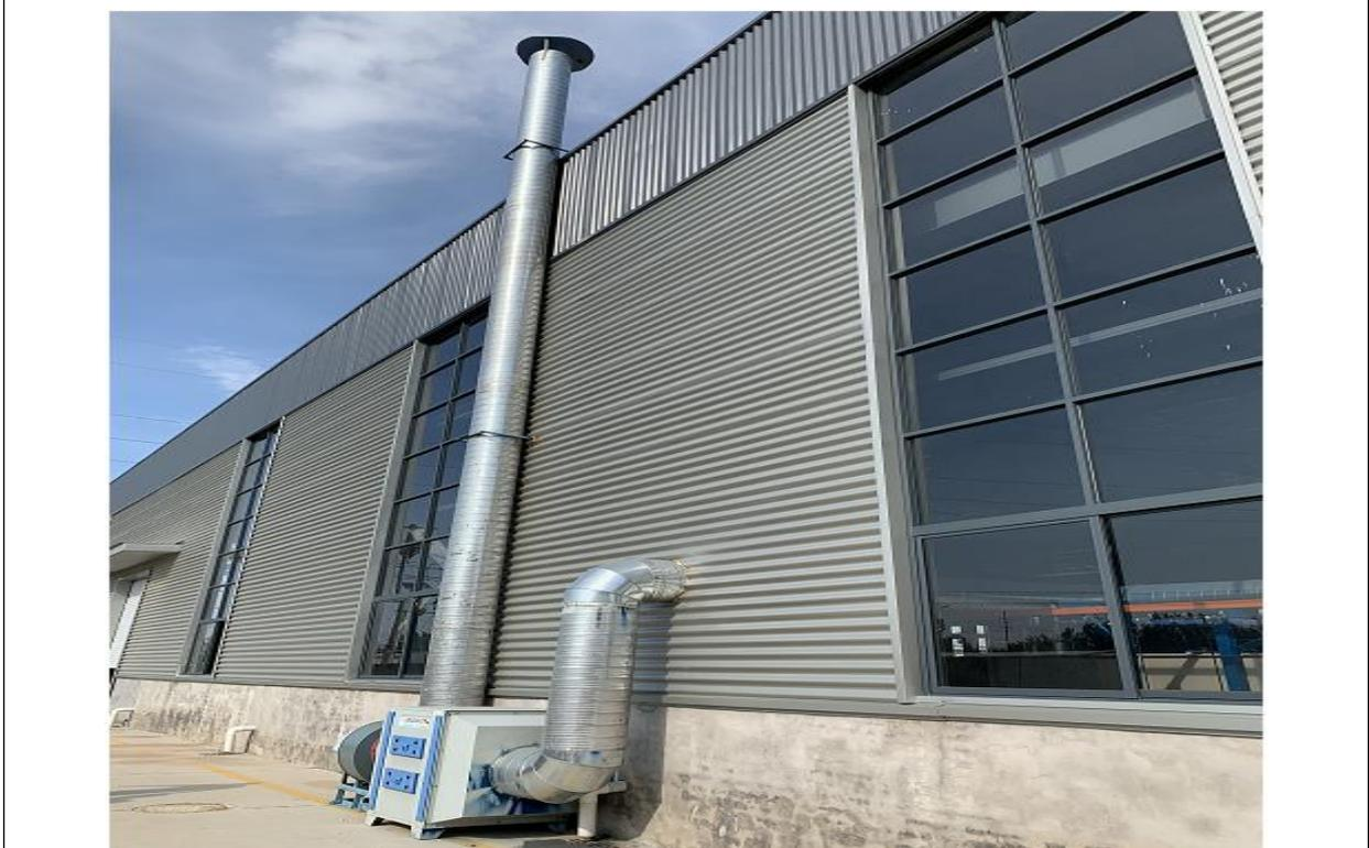
喷漆房：集气罩+过滤棉+二级活性炭吸附装置+15m 高排气筒
